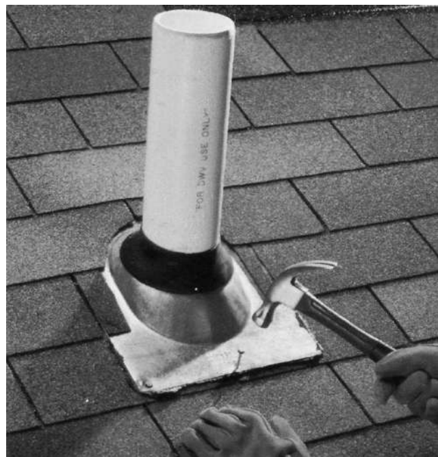
2 Slide the flashing over the vent pipe, and carefully tuck the base of the flashing up under the shingle. Press the flange firmly against the roof deck to spread the roofing cement, then anchor it with rubber gasket flashing nails. Reattach loose shingles as necessary.
