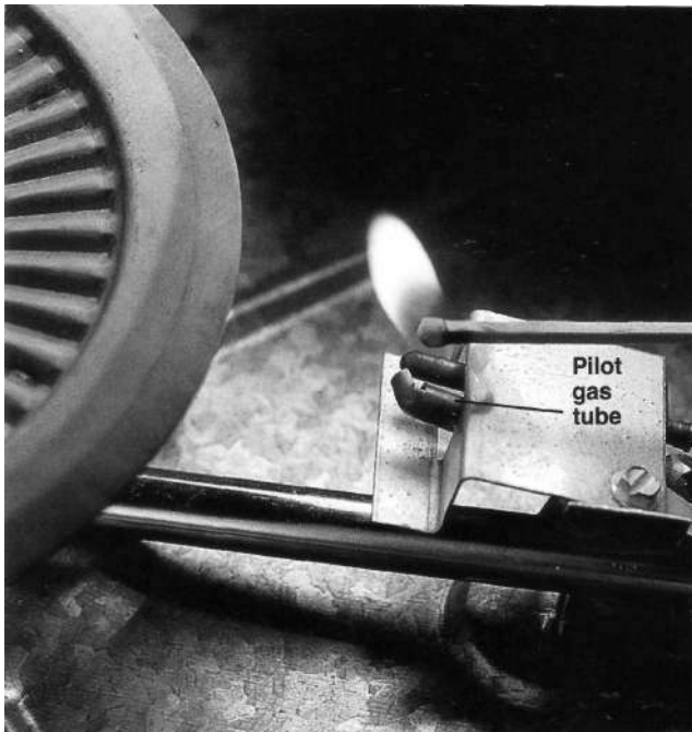
22 Light a match, and hold flame next to the end of the pilot gas tube inside the burner chamber. Be sure to keep your face away from the opening.
