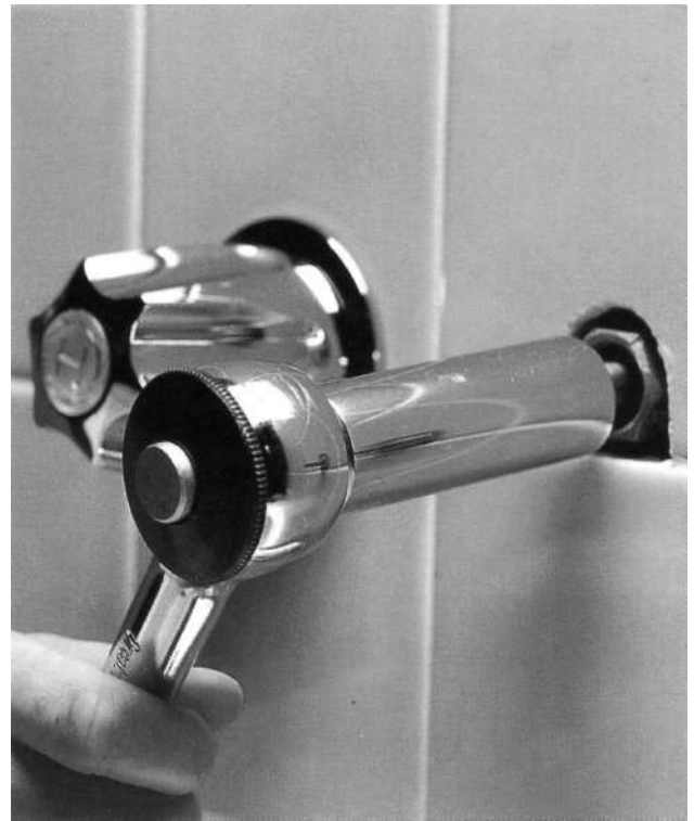
3 Unscrew the stem assembly, using a deep-set ratchet wrench. If necessary, chip away any mortar surrounding the bonnet nut (page 201, step 2).
