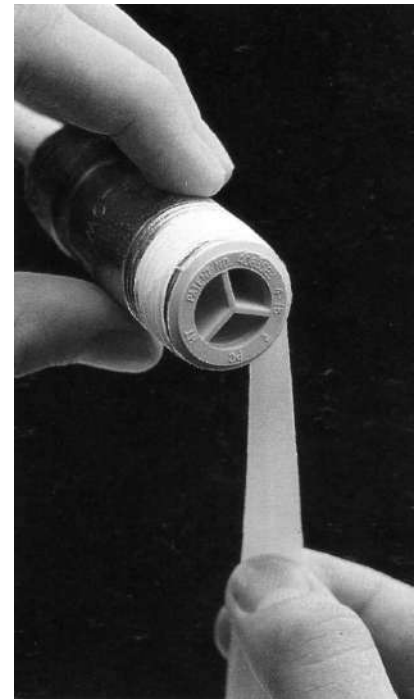
13 Wrap Teflon tape around the threads of two heat-saver nipples. The nipples are color-coded, and have water-direction arrows to ensure proper installation.
