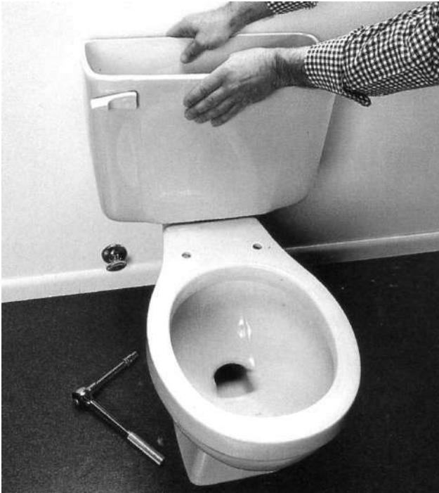
11 Turn tank right side up and position it on rear of toilet base so that spud washer is centered in water inlet opening.
