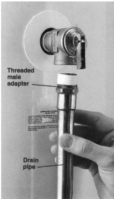
11 Attach a copper or CPVC drain pipe to the pressure-relief valve, using threaded male adapter (page 43). Pipe should reach to within 3" of floor.
