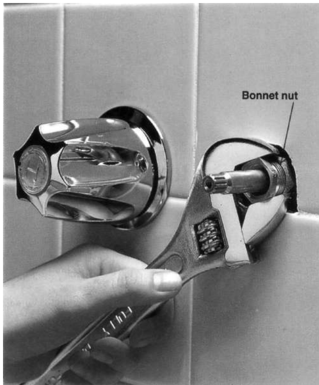
2 Remove bonnet nut with an adjustable wrench or channel-type pliers.
