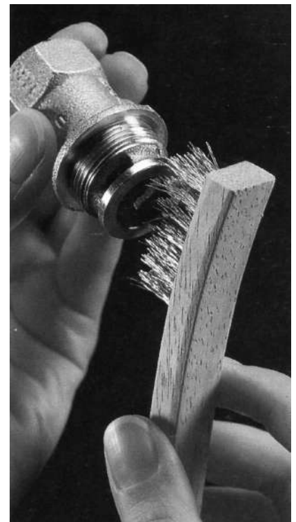
6 Clean sediment and lime build-up from nut, using a small wire brush dipped in vinegar. Coat all parts with heatproof grease and reassemble diverter valve.
