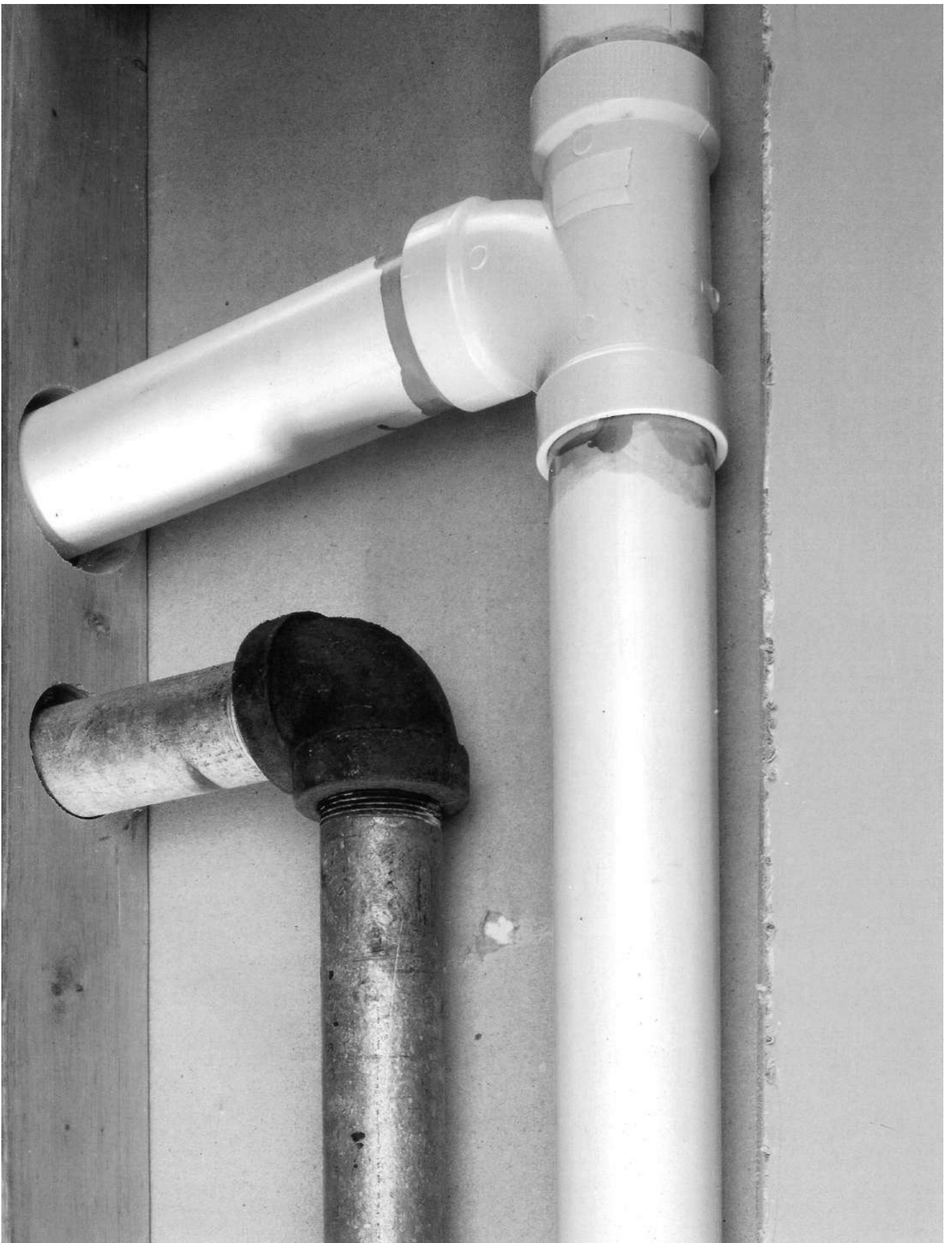
Leave old plumbing pipes in place , if possible. To save time, professional plumbing contractors remove old plumbing pipes only when they interfere with the routing of the new plumbing lines.
